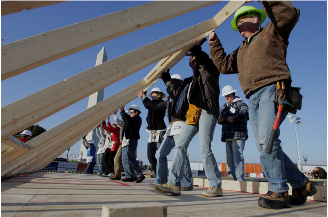
Volunteers raise a wall on a Habitat for Humanity home, Washington, D.C., November 2005. (Photo by Joe Raedle/iStock)
